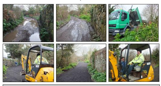
Photos: top row left to right: muddy path in 2016 after lots of rain; path before we started work in March 2017 (after a dry period); tipping the planings; bottom row left to right: spreading the planings; the finished path; A job well done—thanks to Tom and Ken!
